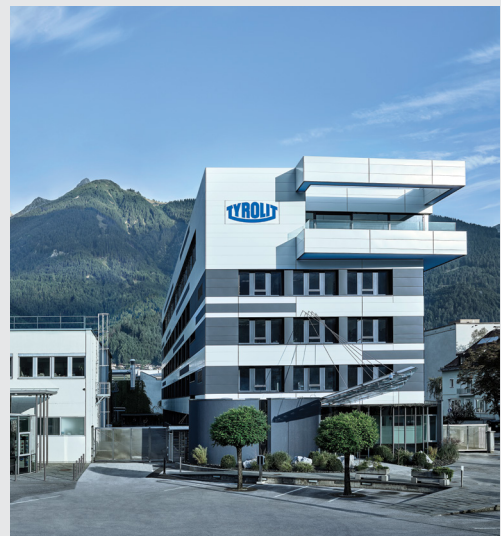
TYROLIT headquarters in Schwaz (Austria)
